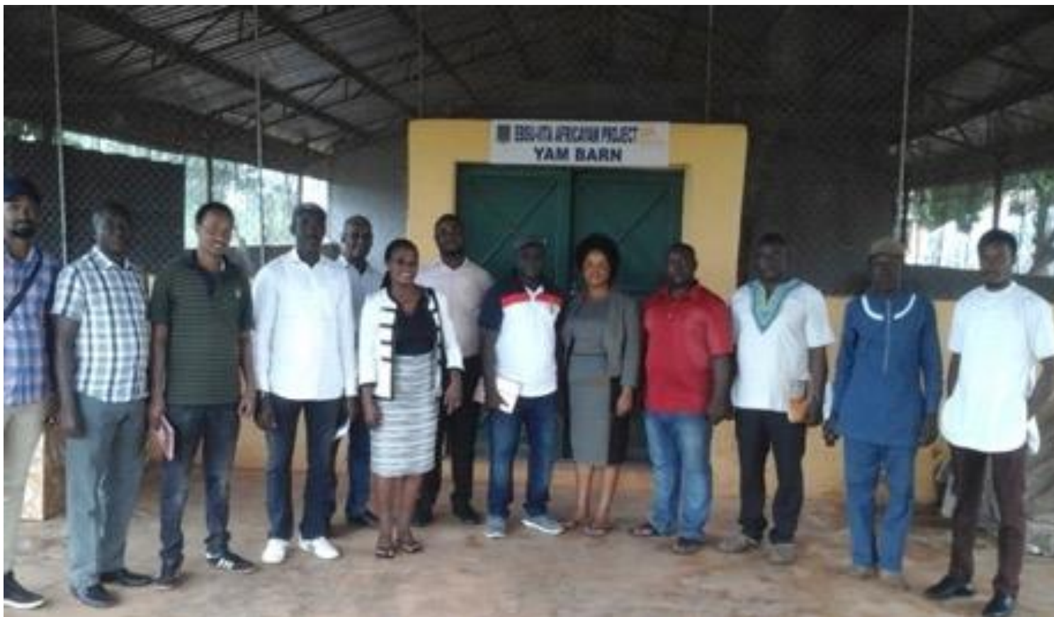
Modern Yam Barn constructed at CAS Campus, EBSU
